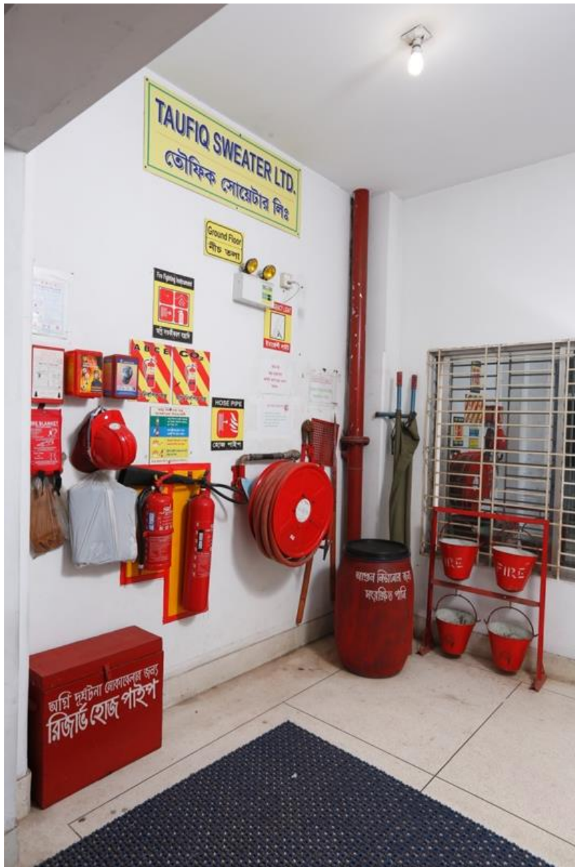
Fire Fighting equipments & Alarm Control Panel
