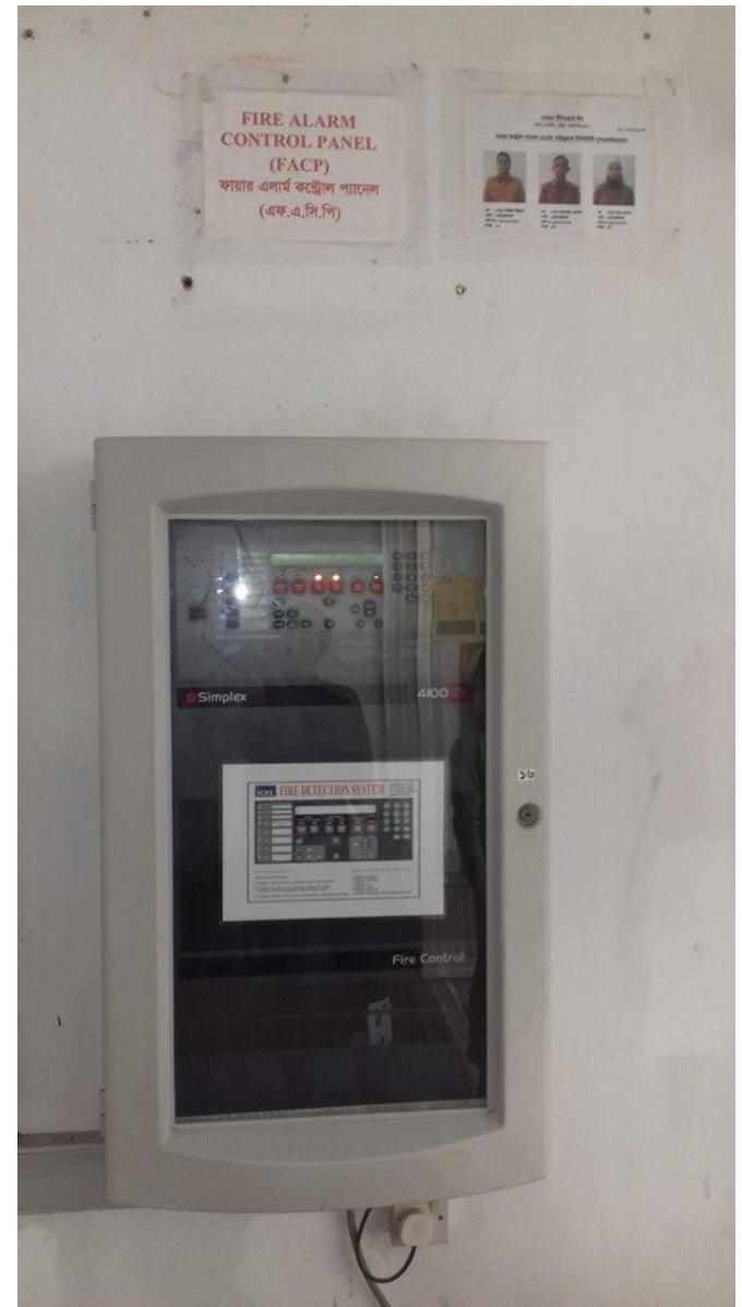
Fire Fighting equipments & Alarm Control Panel
